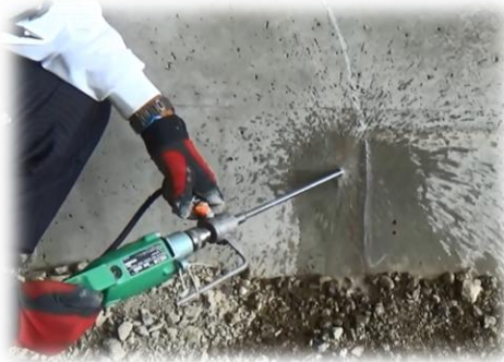
Drilling injection holes using a water jet drill
