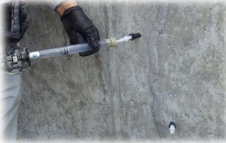
Construction by pressurized injection using a manual injection pump
